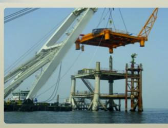
This Deck with the Equipment operates as a Wellhead Deck in which draws the gas from Hengam Field with a pressure, approximately 450 Bar and deliver this to Onshore Facilities to be treated with certain process.
