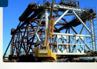
Weight of the Jacket is 1000 Tons and weight of the Piles is 1000 Tons. The Jacket have four legs, six conductors and four elevations.
